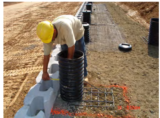
Sleeve-It 1224R installation behind SRW
