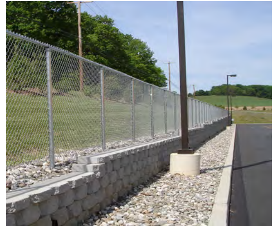
Sleeve-It's Fence Post Integration system installed at the DHL Facility
