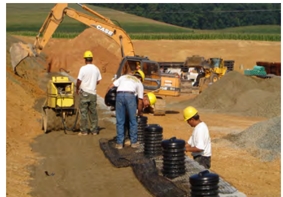
Sleeve-It Product integration with SRW construction
