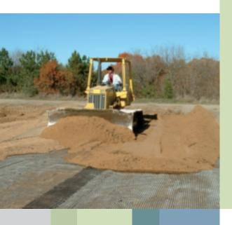
For 30 years biaxial geogrids have been utilized in pavement construction and soil stabilization projects throughout the U.S. and worldwide. StrataBase stabilizes aggregate/soil through confinement and introduces tensile elements, thereby increasing bearing capacity and load support capacity. StrataBase applications include:
