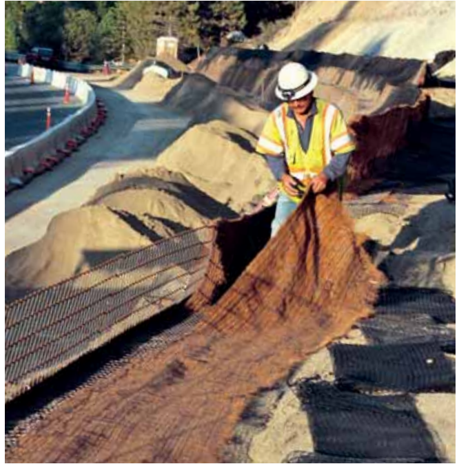
PHOTO 4 As baskets were placed, each was wrapped in a biodegradable coconut blanket to control erosion and stabilize the soil while local vegetation was established on the micro-terraces. The blankets were seeded by hand on the slope-facing side of the blanket.
